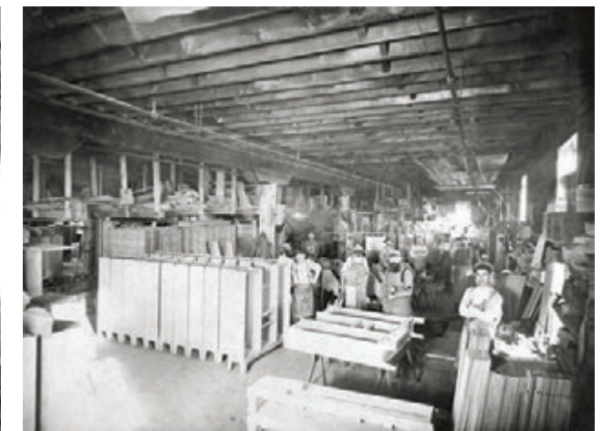
The cabinet shop at Rockford Standard Furniture Company, Rockford, in 1901. Benson Stone Co., Rockford, Illinois
